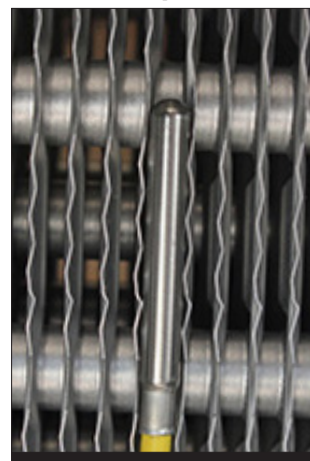
Figure 5 - Option 2: Sensor Positioned Parallel to Evaporator Fins
